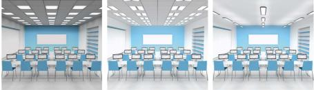
The recessed luminaires with louvers – see the figure 1 – do not provide sufficient illuminance of the vertical surfaces and ceiling. At the same time they represent a risk of arising undesirable reflections on the screens due to the indirect glare. The recessed or suspended luminaires with the direct and indirect characteristic of radiation with diffuse surface or microprism represent an optimal solution
