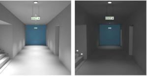
During normal operation the illumination level of communications zones reaches prescribed levels. During the blackout or in case of fire emergency lighting ensures the pupils basic visibility and orientation during leaving the space or to make their access to the fire extinguishers easier.
