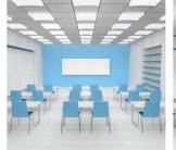
The suspended luminaires with the direct and indirect character of the luminaire MIRZAM with the direct and ninous flux distribution which direct 50% of radiation directly to the task area and 50% towards the ceiling represent an ideal lighting solution for the classrooms. The required distribution ratio of the direct and indirect component of illumination is achieved by placing the luminaire in the distance of 0.3 to 0.6 metre from the ceiling.
