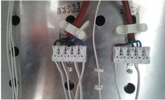
Step 6 :- Plug in gear box and switch on power. Check for correct operation.
